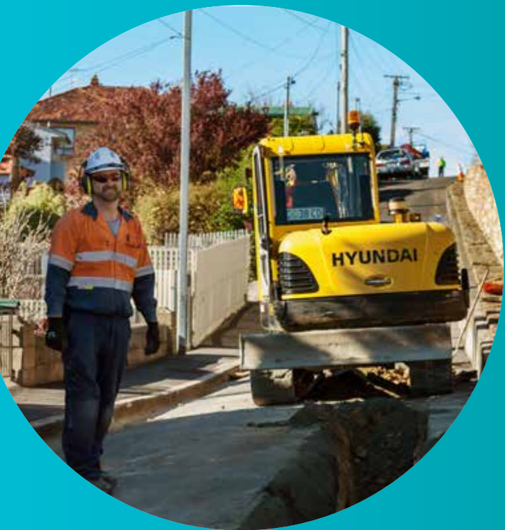
TasWater's Civil Maintenance Plumber, Danny Cleaver, at work in West Hobart.
