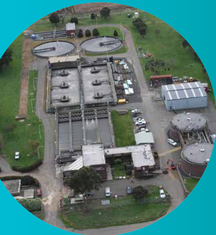
Ti Tree Bend Sewage Treatment Plant is one of the facilities currently servicing the Launceston community.
