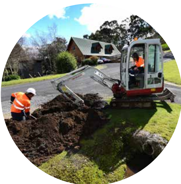
Andrew Hooper and Robert Emery laying new infrastructure in Latrobe.
