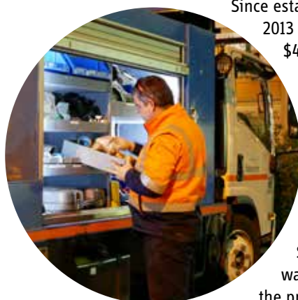
Heath Mayne working on a reticulation pipe repair in Kingston.
