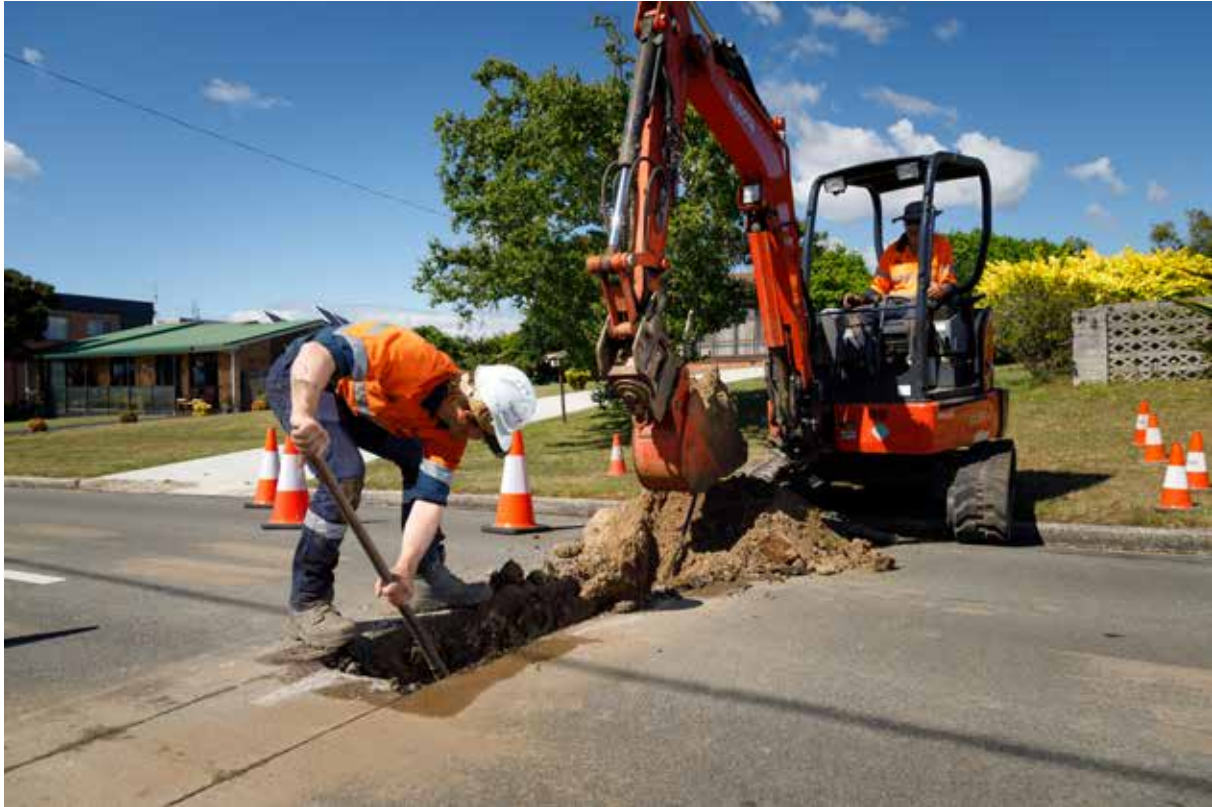
Kane Brooks and Robert Emery undertaking reticulation works in Shearwater.
