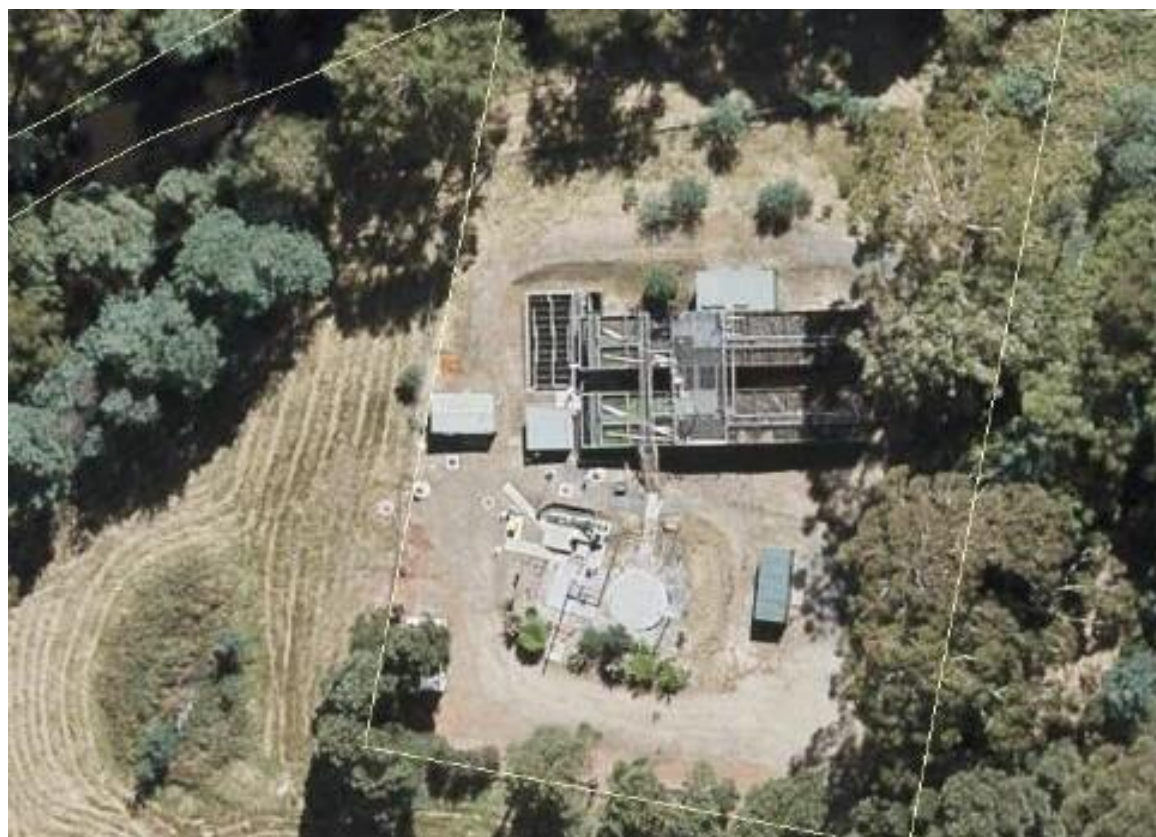
Figure 24-1: Geeveston Sewage Treatment Plant
