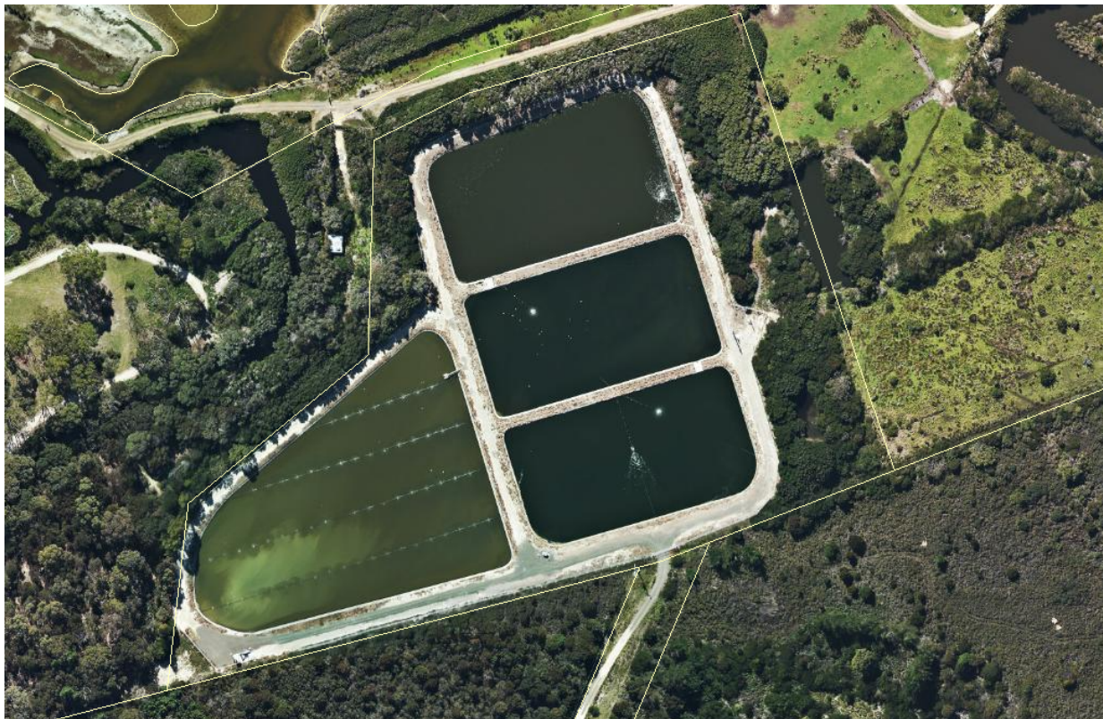
Figure 3--1: Bicheno Sewage Treatment Plant
