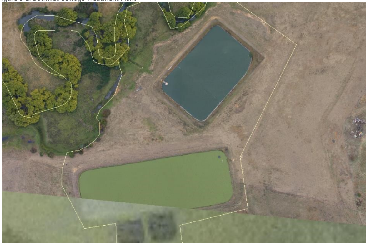
Figure 6-1: Bothwell Sewage Treatment Plant
