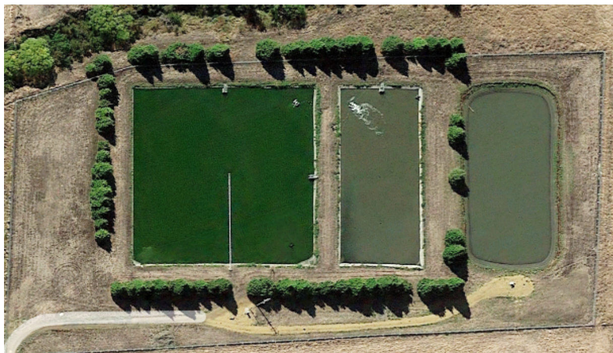
Figure 12-1: Campania Sewage Treatment Plant
