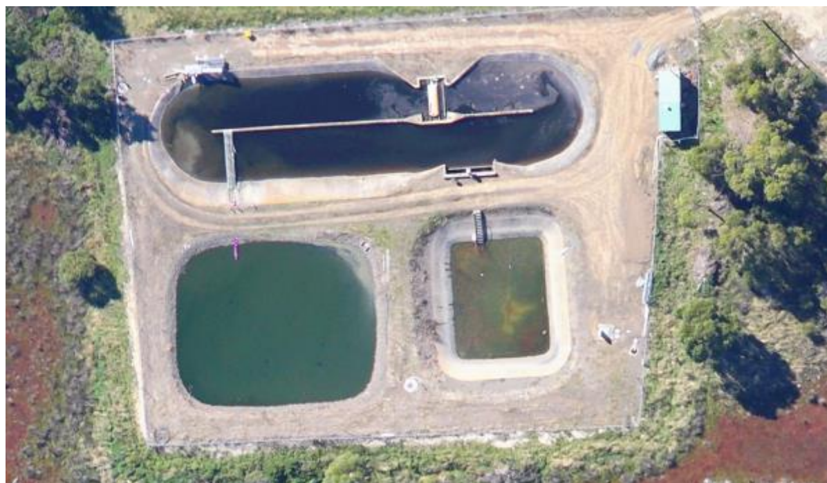
Figure 18-1: Cygnet Sewage Treatment Plant
