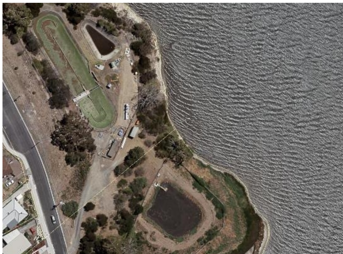
Figure 34-1: Midway Point Sewage Treatment Plant
