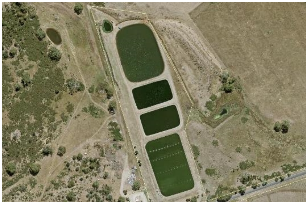
Figure 68-1: Swansea Sewage Treatment Plant
