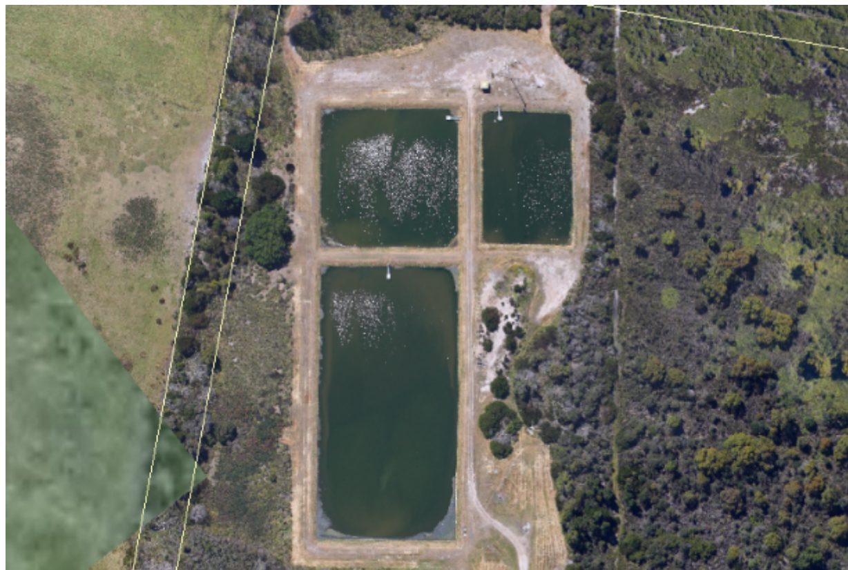
Figure 71: Bridport Sewage Treatment Plant
