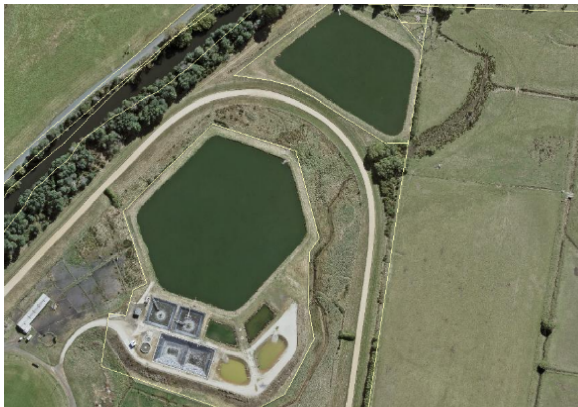
Figure 19-1: Deloraine Sewage Treatment Plant
