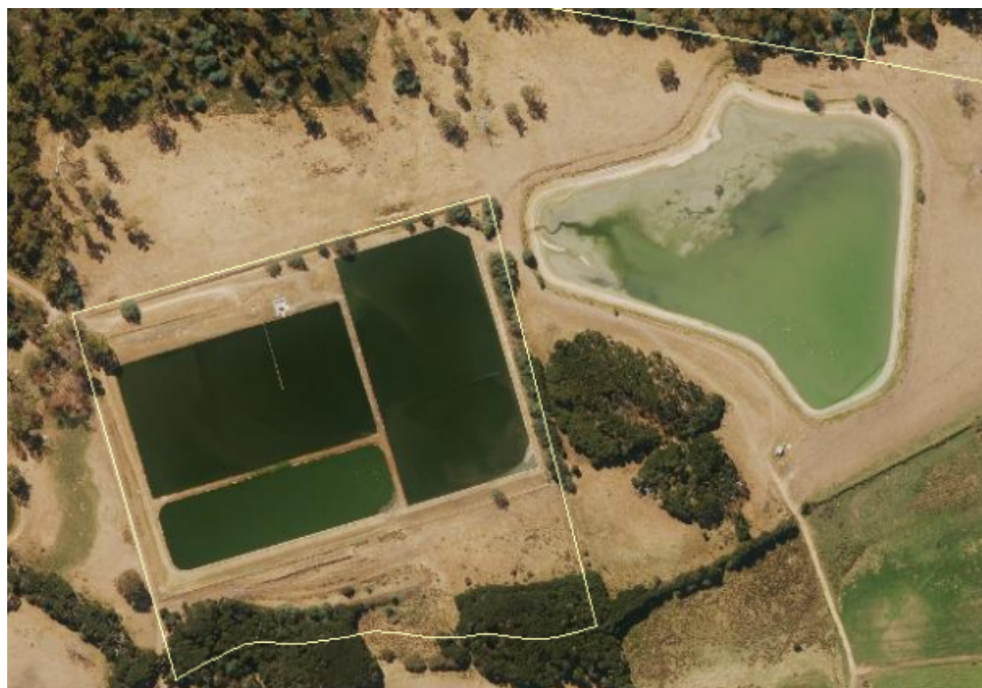
Figure 30--1: Legana Sewage Treatment Plant
