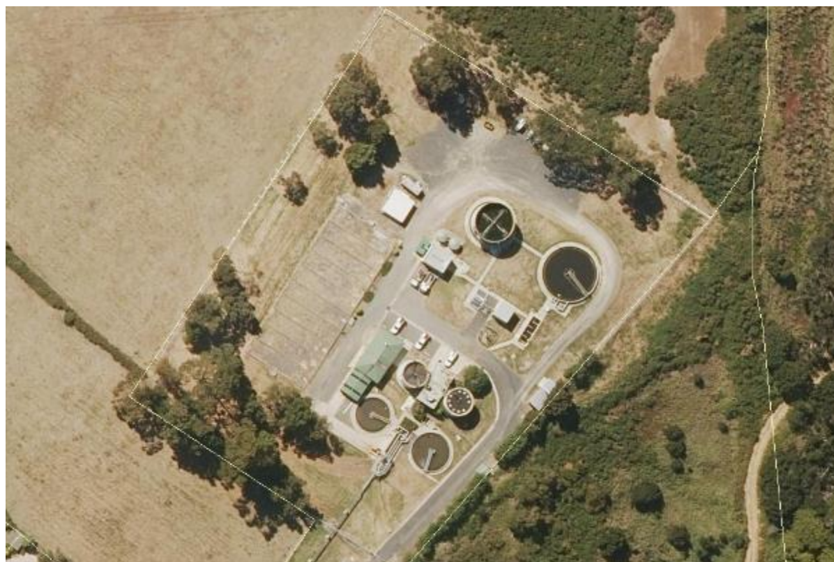
Figure 51-1: Riverside Sewage Treatment Plant
