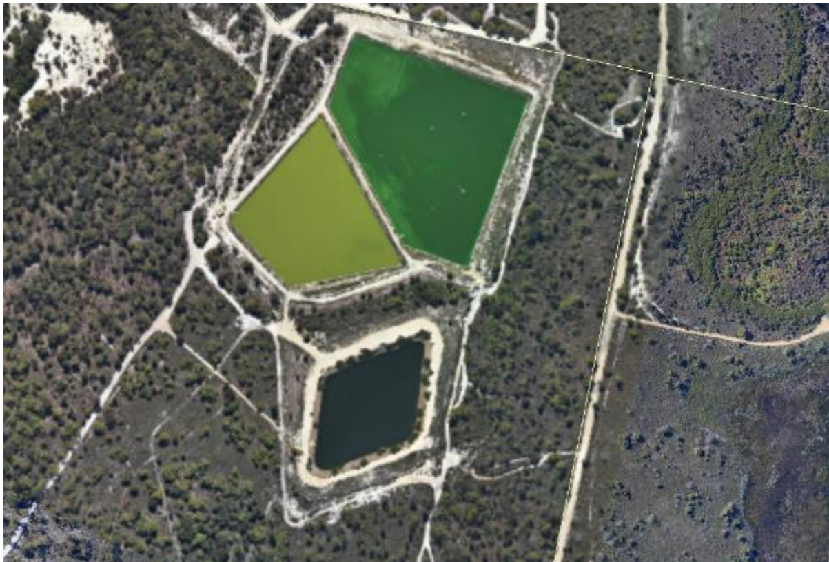
Figure 66-1: Steiglitz Sewage Treatment Plant
