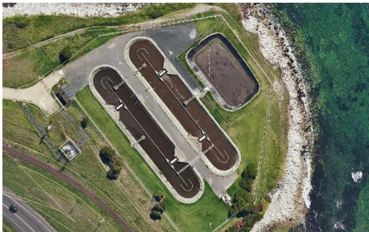
Figure 61-1: Somerset Sewage Treatment Plant
