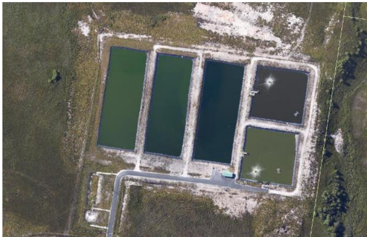
Figure 67-1: Strahan Sewage Treatment Plant
