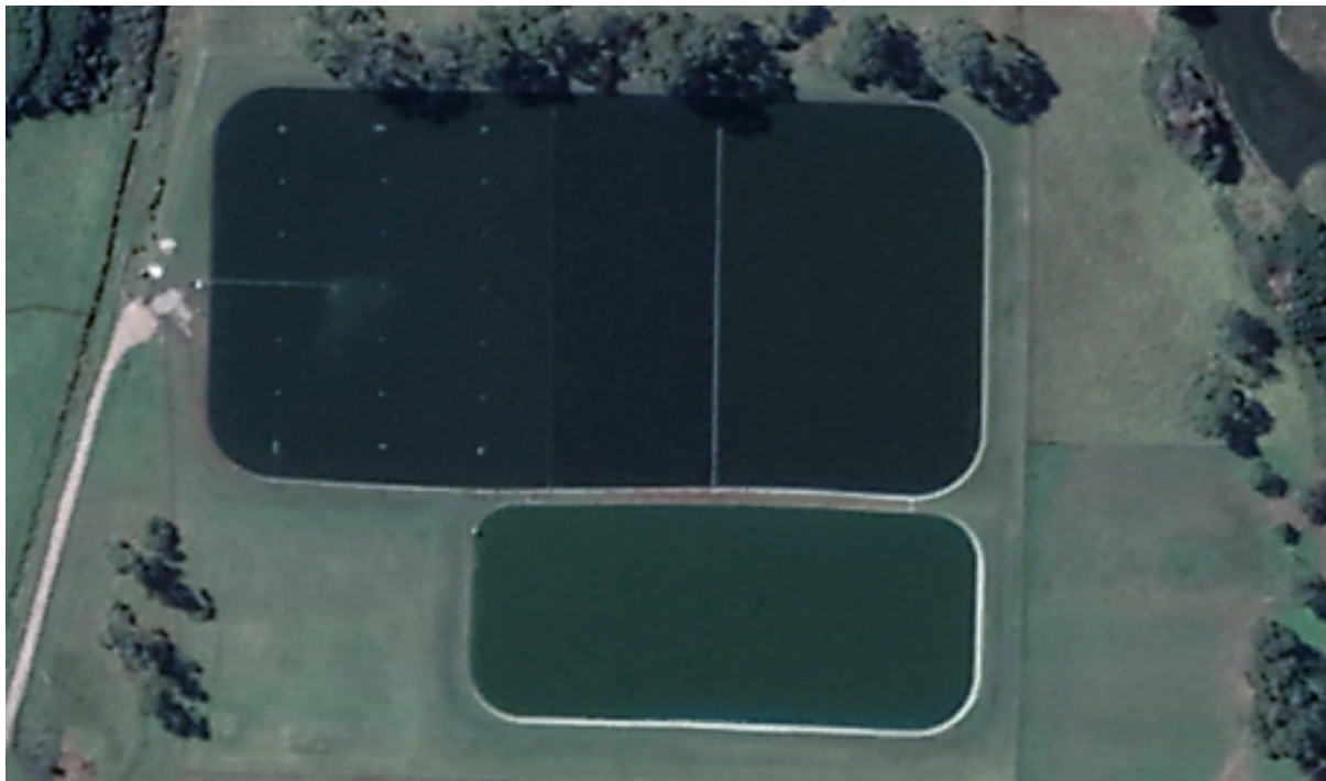
Figure 72-1: Turners Beach Sewage Treatment Plant
